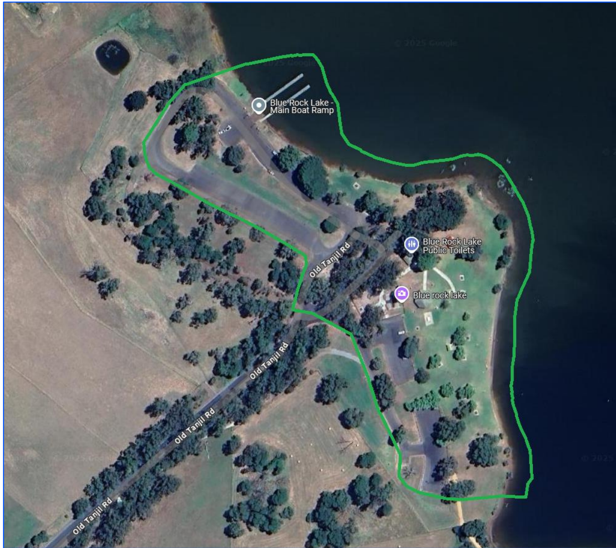
Figure 4: Blue Rock Lake Western Recreational Area (Public access area, excluding boats, delineated in green and in approximate terms). Source: Google Maps
