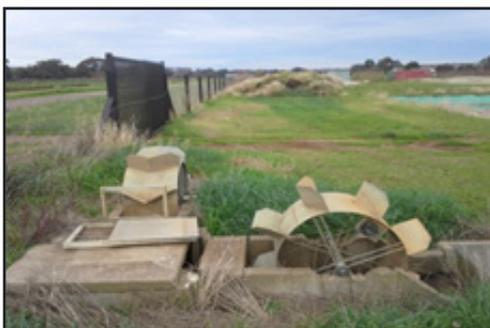
Most deliveries are through old inaccurate Dethridge wheels. These generally under-record deliveries to customers
