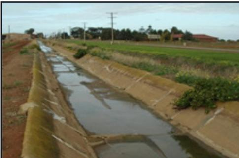
Cracks within the concrete lining the channel supply system let water seep into the ground.
