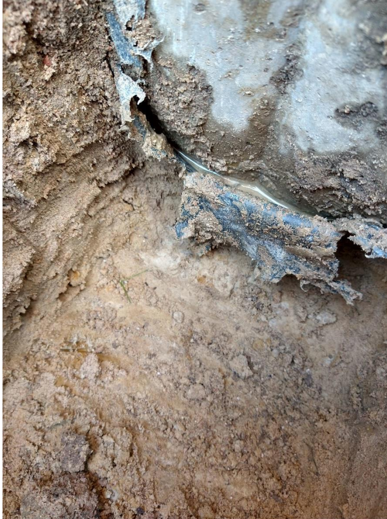
Photograph 2: Base of Silty Sand layer Against Slab Footing
