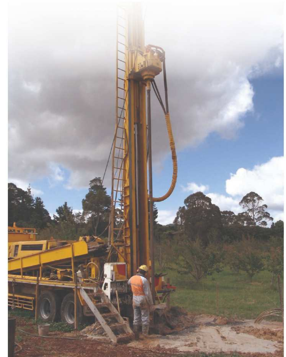
State observation bore drilling at Hawkesdale
