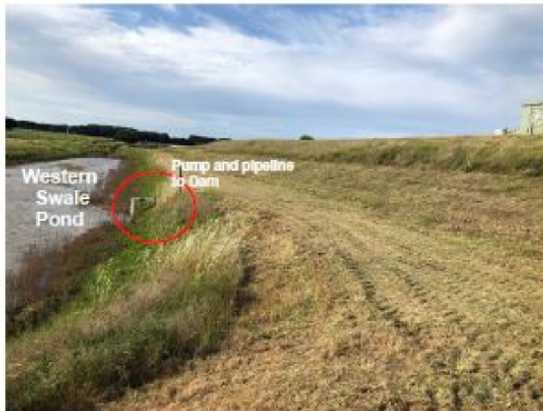
Plate B14: Western swale pond. Below ground excavation capturing surface water runoff from paddocks. Water is pumped into the dam (to the right).
