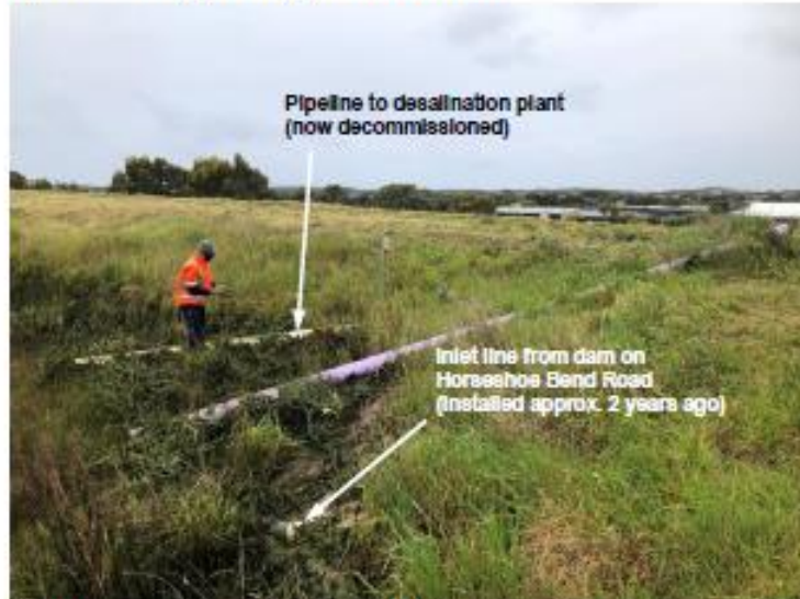
Plate B23: Two pipes pass through the crest (upstream to downstream) at the south-west corner (lowered reservoir on Monday 5 th October 2020).
