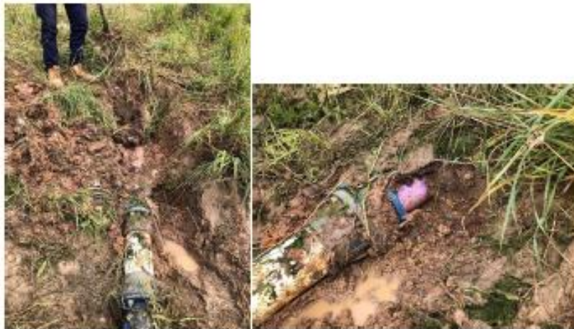
Plate B27: Part length of pipe exposed. Pipe on a slight upslope in line heading toward crest. Loose and wet earthfill around pipe.
