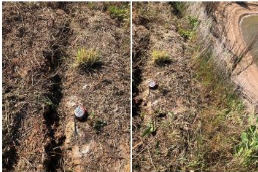
Plate B38: Western embankment section toward the northern embankment. Longitudinal cracks along upstream edge of crest up to 100 mm wide. Coincident with bulge shown in Plate B38. No sign of recent movement.
