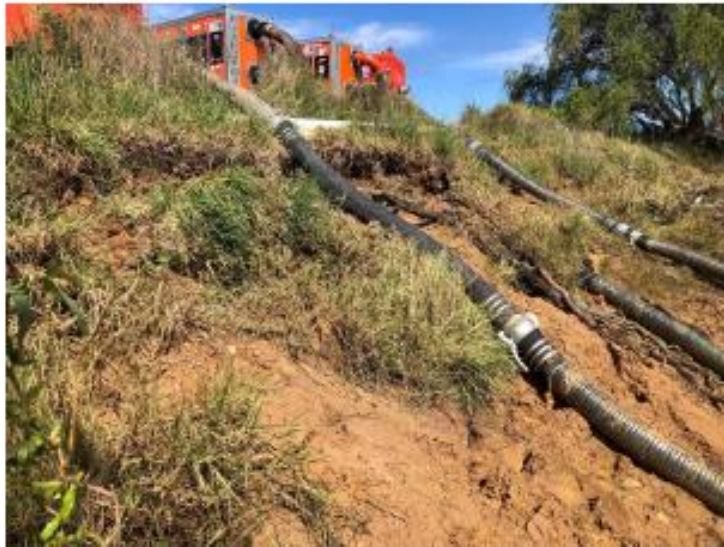
Plate B34: Southern end of eastern embankment. Shallow clumping in upstream shoulder. Assessed as mostly pre-existing drawdown with recent topping of steeper upper bank.
