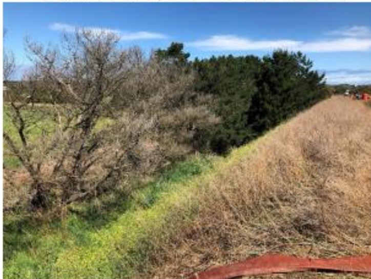
Plate B35: Eastern embankment downstream slope and toe region noting proximity of pine trees to the toe and the group of approx. 8 dead trees.
