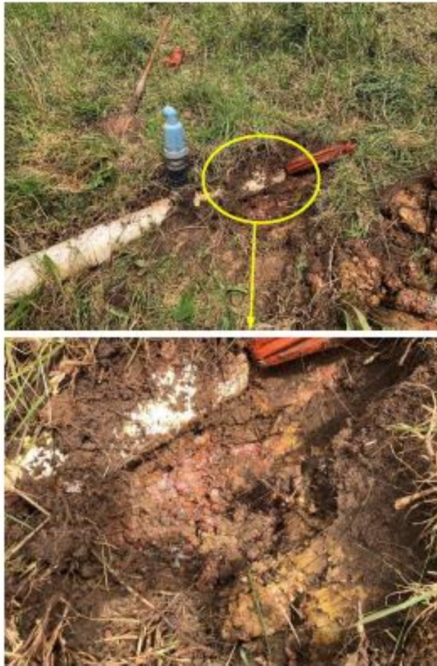
Plate B26: Part length of decalcification pipe exposed with plastic marker sheet on top of the pipe. The earthfill was in moist condition around the pipe. No seepage observed from earthfill. Pipe was near horizontal within earthfill.
