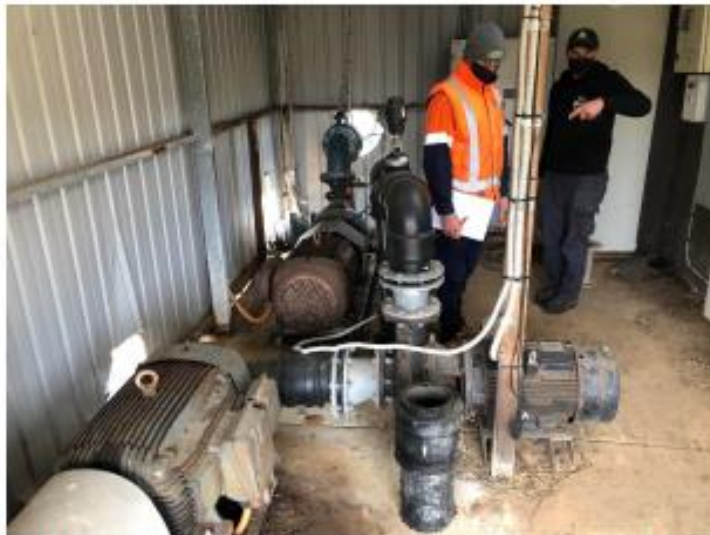
Plate B17: Inside the pump shed. Foreground and left is the pump for the northern irrigation line, middle pump is to the golf course and top pump is to the dam is the property to the west.
