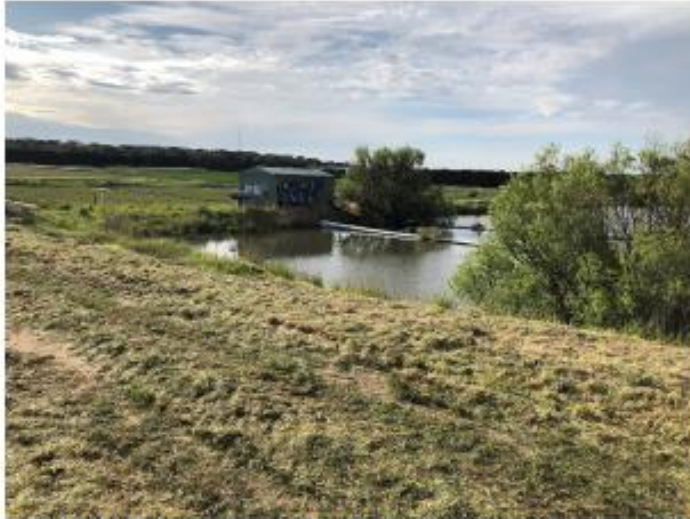
Plate B7: South-west corner of embankment (4 pm Saturday 3 rd October 2020). Reservoir level had been drawn down at least 0.2 m by this time. Pump shed on western bank and this is close to the low point in the crest.
