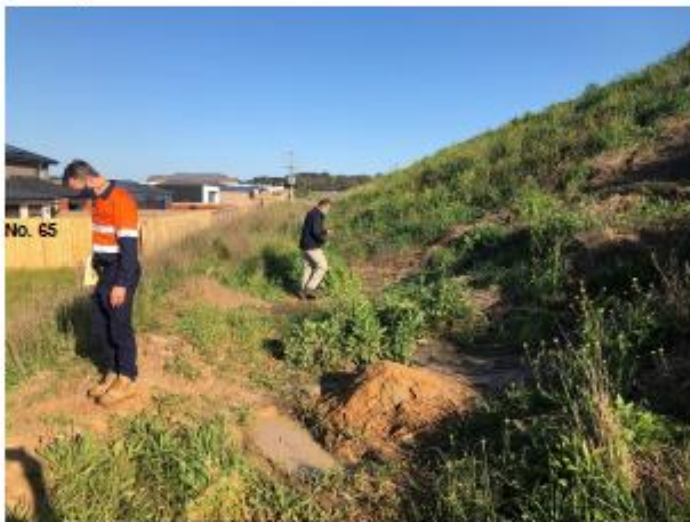
Plate B8: Downstream shoulder and toe of southern embankment looking west (7:30 am Saturday 3 rd October 2020). Pooled water in holes dug for bike jumps.
