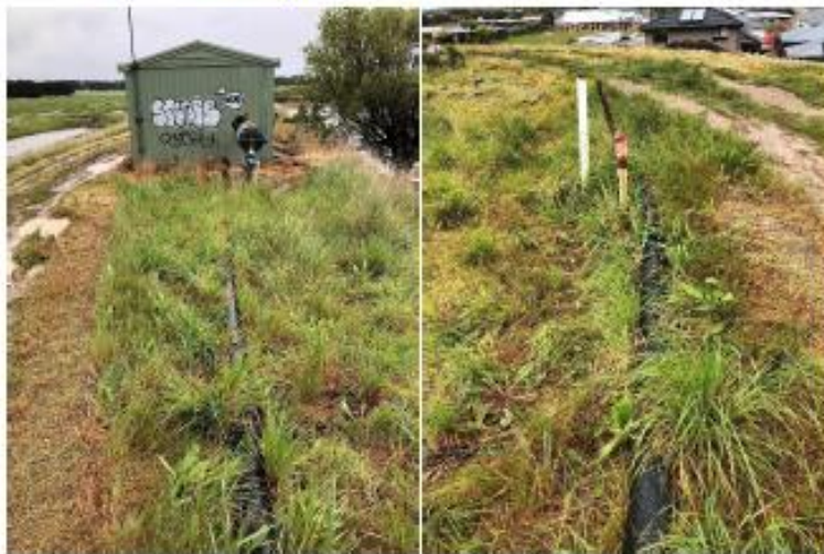
Plate B22: Inlet / outlet line to the golf course located on surface of crest. Extends below ground a short distance past the pvc pipe (right) and then crosses the crest of the southern bank down the downstream face to the golf course.
