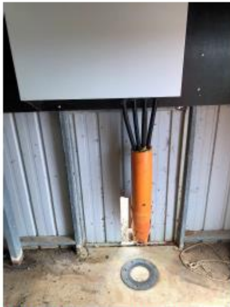
Plate B21: Power entry on western side of shed. Power lines extend below ground along the western bank crest and down the ramp to the power pole shown in Plate B20.
