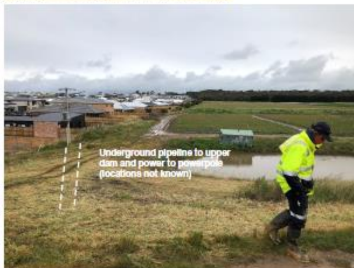
Plate B20: (Top) Southern outlet line exits the shed and then extends below ground along the upstream edge of the western bank crest (the pipe with the red cap is an air release valve on the pipe). (Bottom) The pipe is understood to head down the ramp and connect into the pipeline running along the site boundary (pipeline from treatment plant to upper dam).
