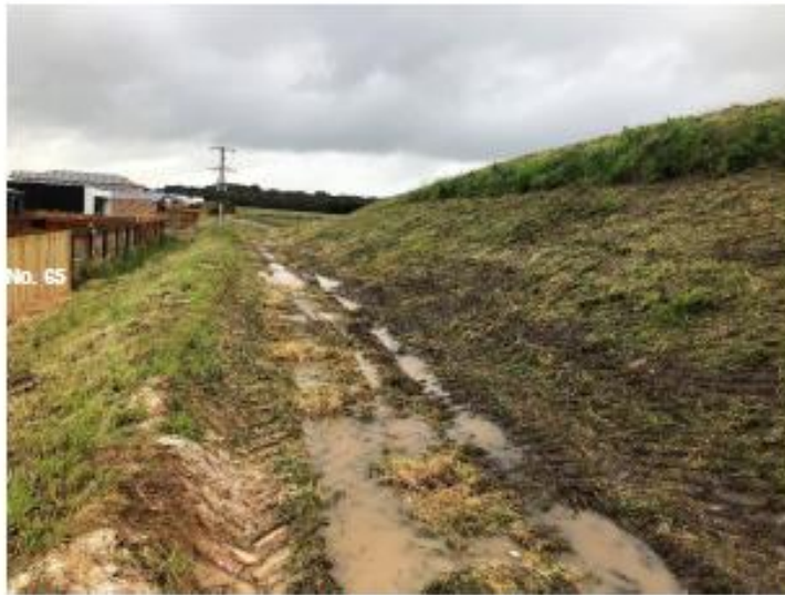
Plate B18: Downstream shoulder and toe of southern embankment looking west, after rainfall (8:30 am Monday 6 th October 2020). Pooled water in swale.
