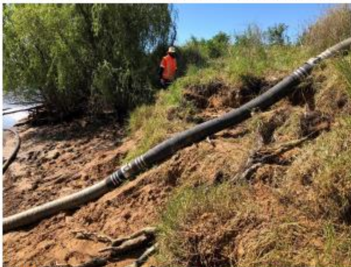
Plate B33: Southern end of eastern embankment. Shallow clumping in upstream shoulder. Accessed as mostly pre-existing drawdown with recent toppling of steeper upper bank.
