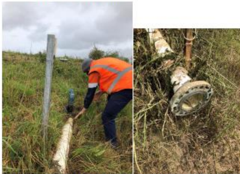
Plate B24: Desalination offtake pipeline that was at reservoir level on Saturday 3 rd October 2020. End flange (right) is not closed off (tape extended full 8 m within pipe). Pipe extends through the embankment crest approx. 1 m below crest level.
