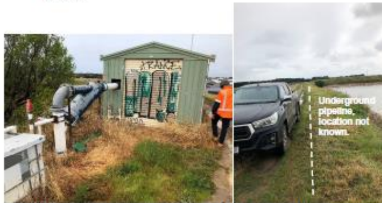
Plate B18: (Left) Northern Irrigation line exiting mid height from the shed and then entering the ground. (Right) pipe extends below ground along the upstream edge of the western bank crest, crossing the crest at the north-west of the dam.
