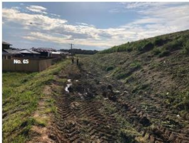
Plate B8: Downstream shoulder and toe of southern embankment looking west (4 pm Saturday 3 rd October 2020). Pooled water from water filled holes.
