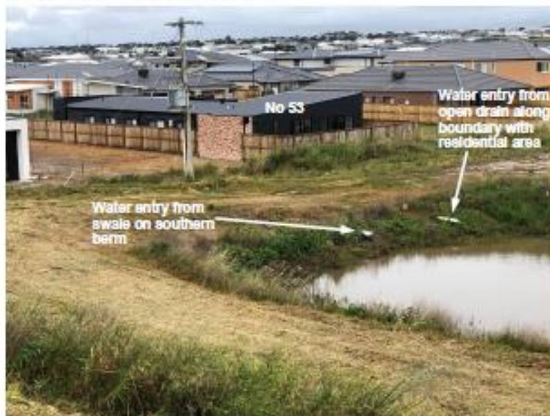
Plate B15: Surface water entry into western swale pond on residential side. Overflow of swale pond would flow south into the residential area.
