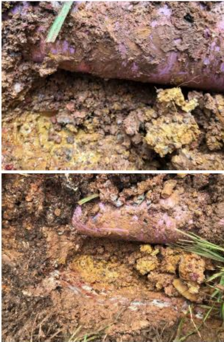
Plate B28: The earthfill was wet and soft around the pipe, very loose below the pipe and seepage was observed. Assessed as poorly compacted around the pipe at this location.
