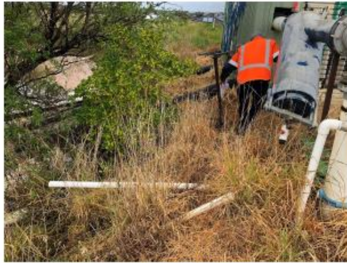
Plate B18: Above ground inlet lines (3 of) from the dam to the pump shed. These connect to the floating pipes shown in Plate B18. PVC pipe in foreground is pressure relief to the northern irrigation line (Plate B18).
