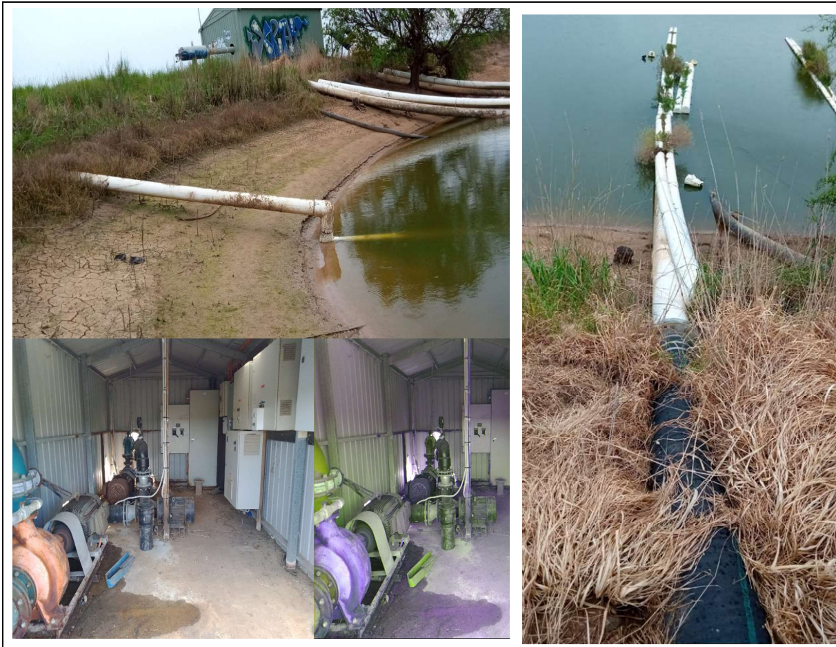
Plates 1 and 2: Inlet and Outlet Pipes and Pump House Arrangement
