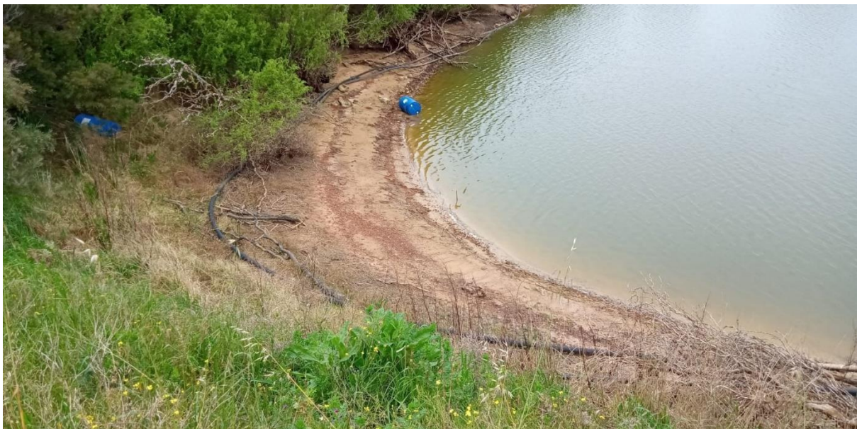
Figure 12 Northeast bank – Black Pipe for erosion reduction of Wave Action
