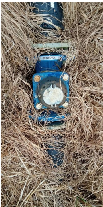
Figure 4 Water Input from golf course flowmeter installed
