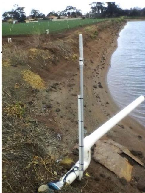
The groundwater team are introducing a new technology to read groundwater meters. The proposed system comprises a low cost, low power transmitting device that is attached to existing water meters and allows hourly data to be sent digitally via radio technology to high-sensitivity receivers. The data is then available to be viewed on-line and quickly and easily imported directly into our metering system.
