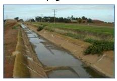
Cracks within the concrete lining the channel supply system let water seep into the ground.
