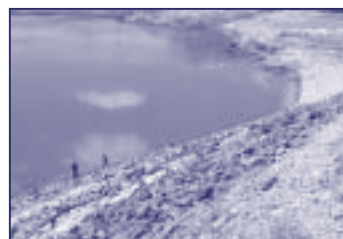
Rock beaching works at Pykes Creek Reservoir
