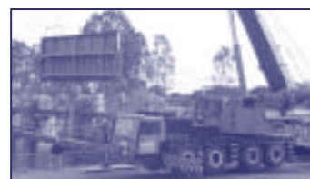
Replacement of gates at Maffra Weir
