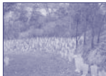
Rehabilitation work at Little Weir
