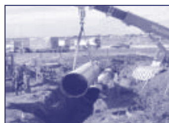
Installing a new pipeline in the Werribee Irrigation District
