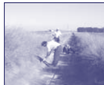
Patching concrete channels in the Bacchus Marsh Irrigation District
