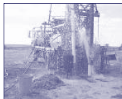
Drilling for groundwater
