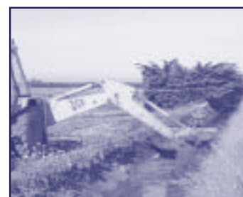
Removing weeds from a channel in the Werribee Irrigation District
