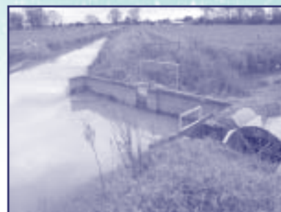
Irrigation channel and water wheel in the Macalister Irrigation District
