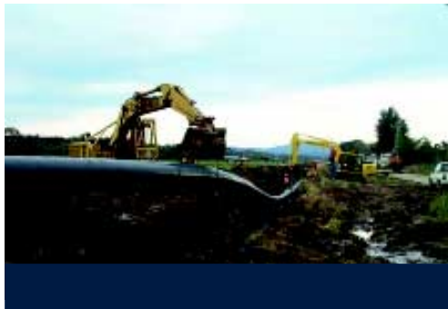
■ Nuntin pipeline project
